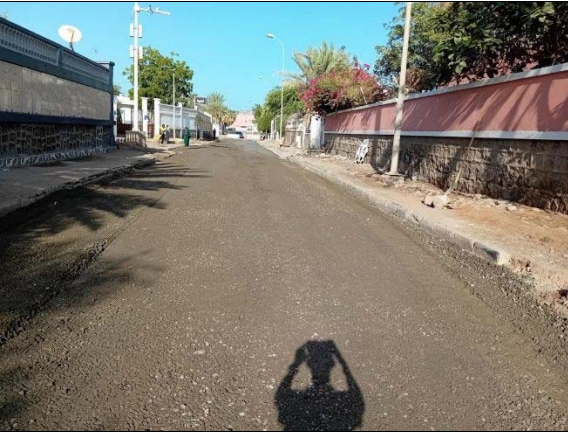
After laying Base-course
