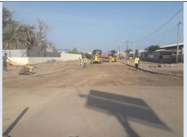
After removal existing pavement
