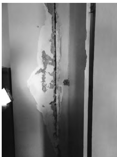
(c) 棟間部の緩衝材
