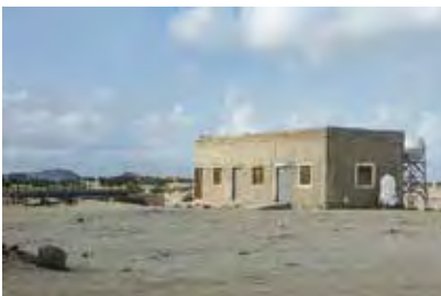
Zula CFC. Roof, windows and doors were renovated
