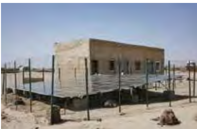
East-south side view
