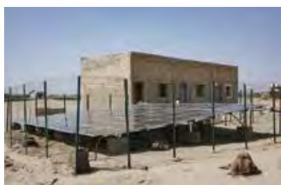
32 pcs of solar panels installed and fenced in Zula CFC
