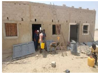
Fig 6-55 Restoring and extending windows and doors
