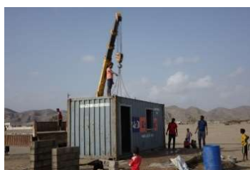
Fig 6-58 Installation of the modified container by MMR Engineering Division staff.
