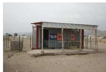
Fig 6-59 Front of the CFC with eaves and concrete poured to create a working area.
