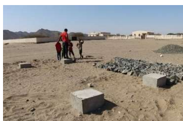
Fig 6-57 Concrete foundation for container installation
