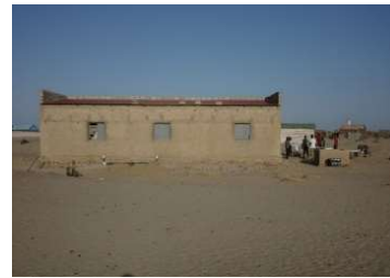
Fig 6-56 Roof replaced and painted, 3 new windows on rear exterior wall
