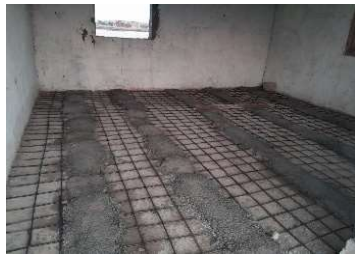
Fig 6-54 Reinforced concrete being poured in ice block machine room floor.
