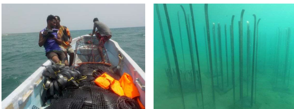
Fig 6-74 C-lant installing operation and it's installed on the seabed.
