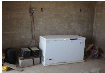
Fig 6-60 Solar-powered freezer installed in Zula CFC for fish storage
