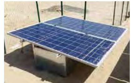
Solar panels installed in Zula CFC
