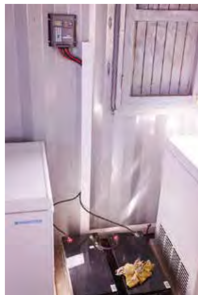
Installation of MPPT controller and batteries
