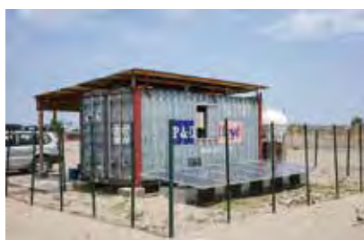
Hirigigo CFC. Modified container house with windows, door and roof
