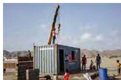
Installing modified container
