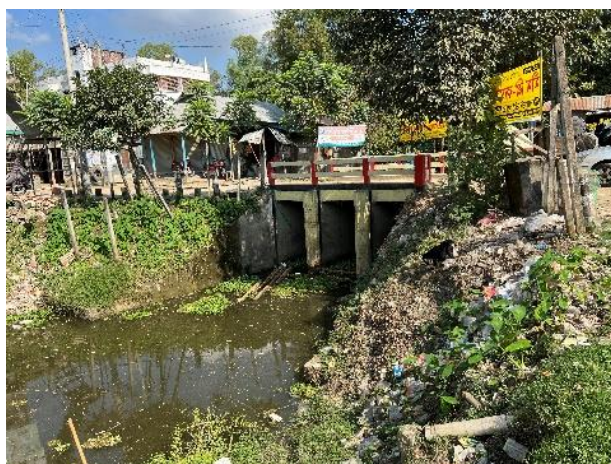
Example of an irrigation and drainage facility (regulator) constructed in a sub-project of Phase 1
