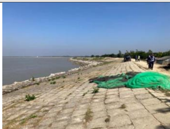
Embankment of Sangu River
