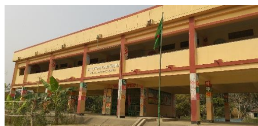
Constructed Multi-purpose cyclone shelter at Debpur, Kalapara Upazila (after Project)
