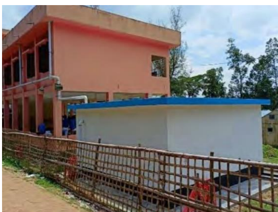
Photo 3.4.1 CHB-made Large-scale Rainwater Tank at a Highschool
