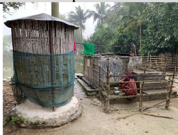
Dug well and sand filter
