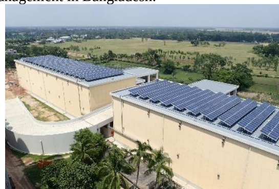
Truck ramps for loading and unloading and solar panels for power generation
