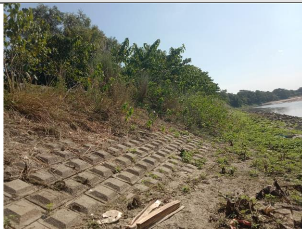
Constructed Embankment in the Pilot Project
