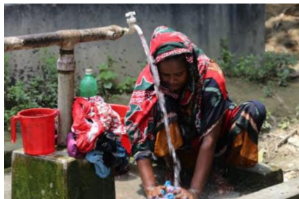
Small-scale piped public water supply facilities in Ghazipur district
