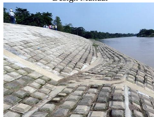
Slope Protection of Embankment at Pilot Project Site
