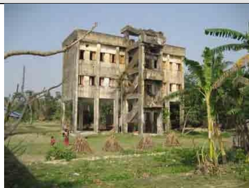
Cyclone shelter at Debpur, Kalapara Upazila (before Project)
