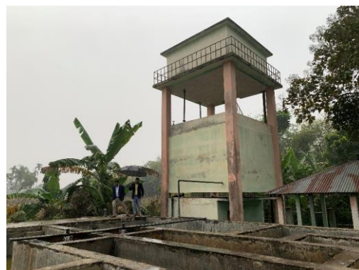
Photo 3.4.5 Well-maintained Arsenic Iron Removal Plant
