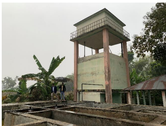
Pipe water supply system
