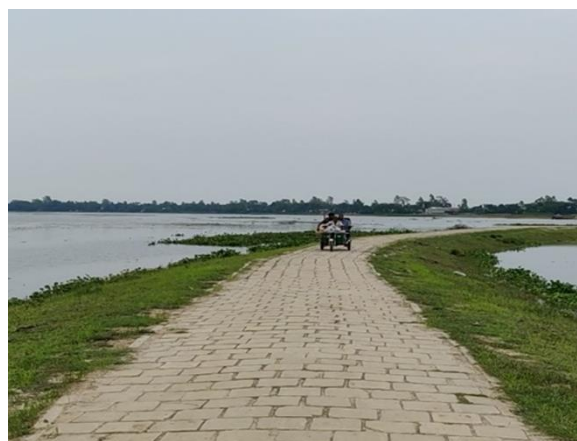
Constructed submersible embankment
