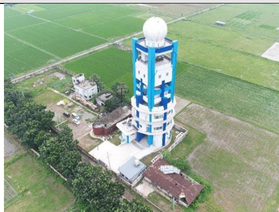
Overview of the Dhaka (Joydevpur) radar tower building
