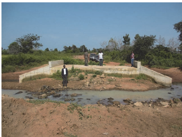
River crossing works under construction by BRD
