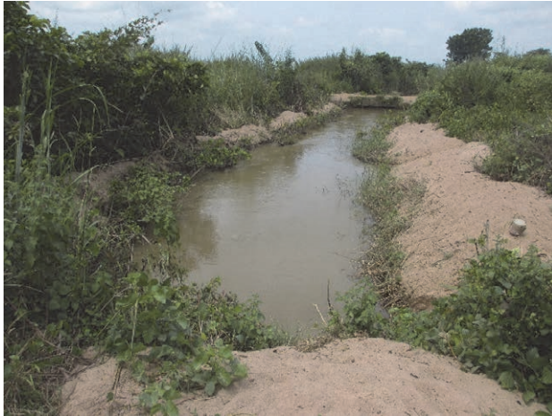
WUA dredging the main canal
