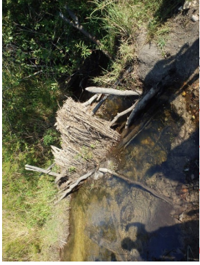
Damaged simple weir shall be repaired.
