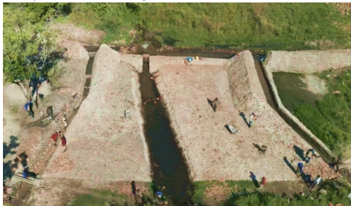
Completion of Permanent Weir Construction (Kasempa District, North-Western Province)
