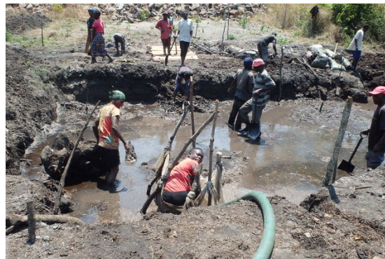
Excavation Work at the Apron Area (Mkushi District, Central province)
