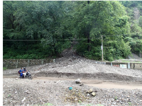
Site conditions in August 2017
