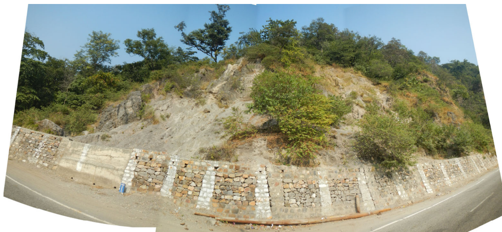
Photo 3.3 Steep slopes (Slope No. 1 (left), Slope No. 2 (right))
