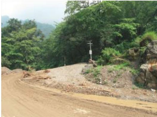
Site conditions in August 2014
