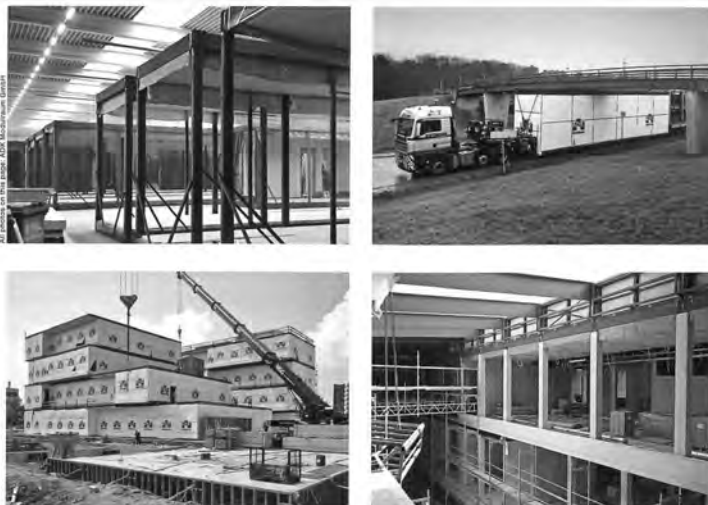
modular construction process
