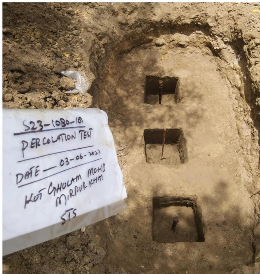
Figure A-3: Percolation test in progress
