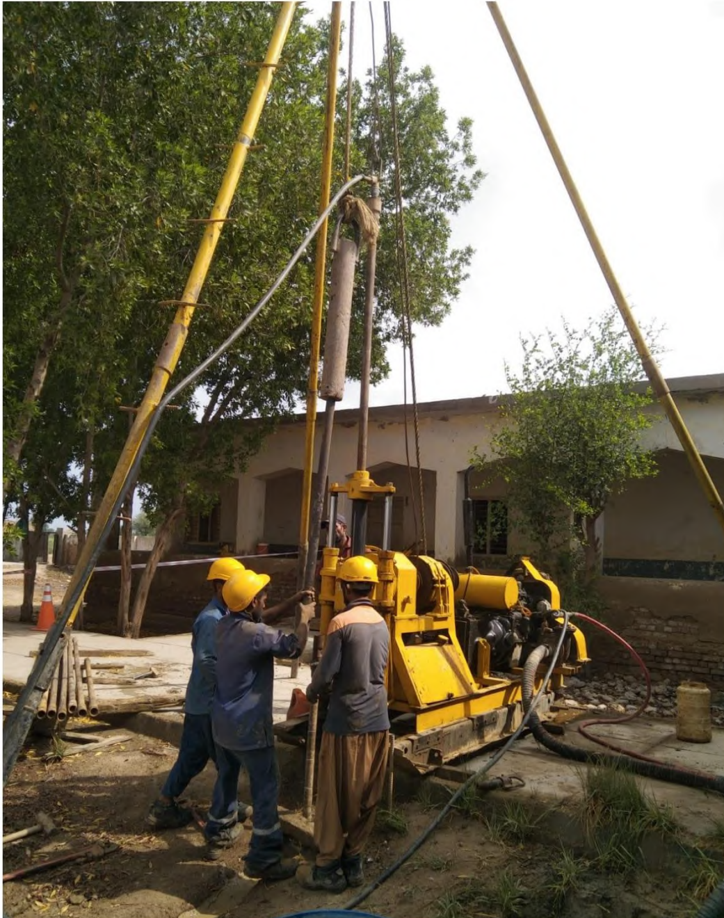
Figure A.2: Performance of Standard Penetration test in progress
