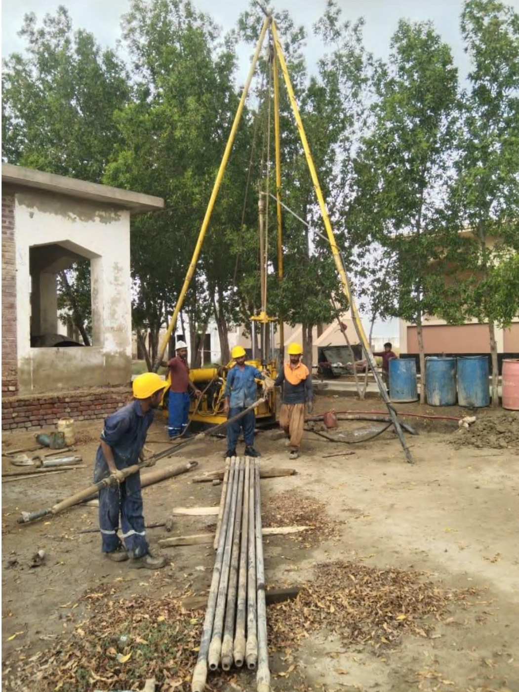
Figure A-1: Drilling works in progress
