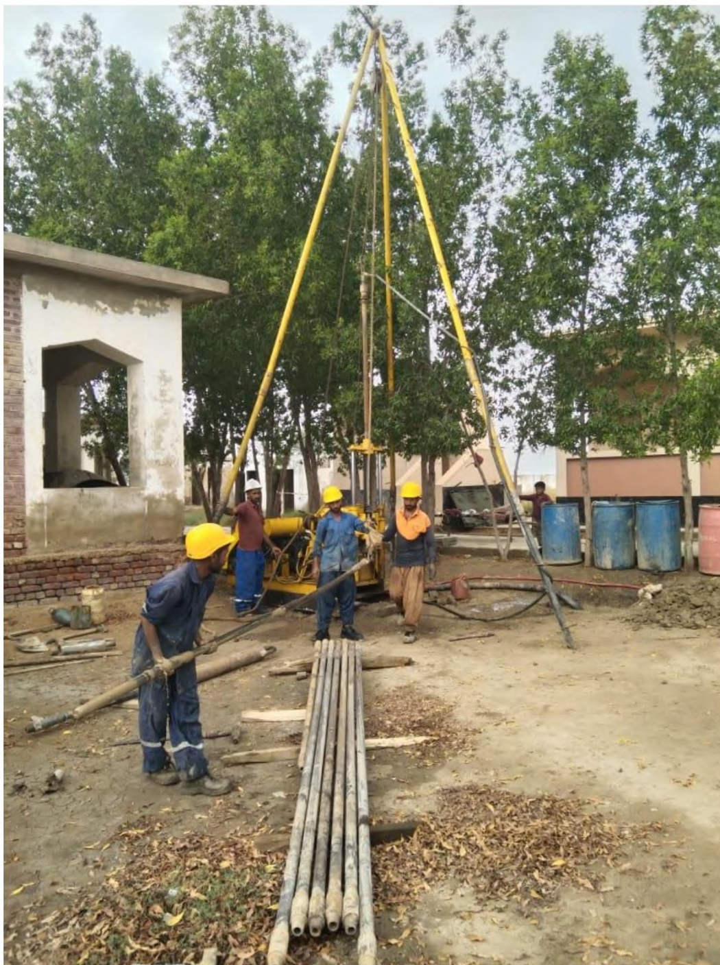
Figure A-1: Drilling works in progress
