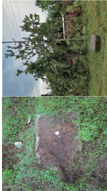
Photo 11 and 12: Telekom manholes
