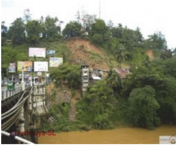
Figure 2-3: Slope failure occurred in Peradeniya
