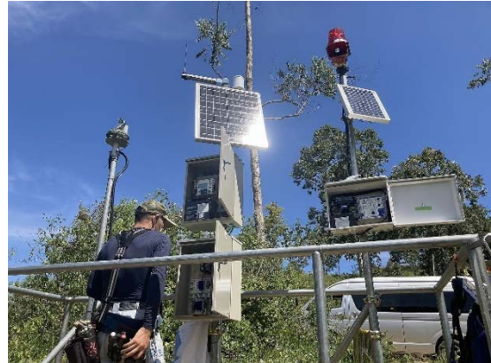
Installed landslide remote monitoring system in Weeriyapura, Badulla on January 25, 2022
