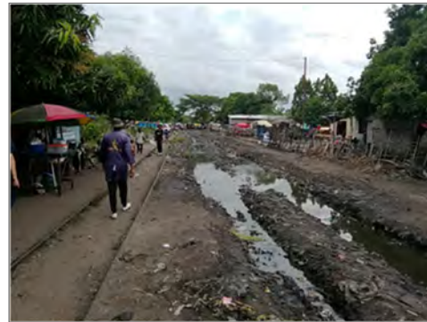
Figure 4-22 Poor Drainage (Approx. 9 k 000 m from Limete Station)
