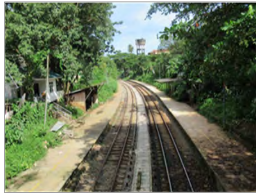
Figure 4-72 After Construction of a Drainage Channel between Tracks (Double Track)
