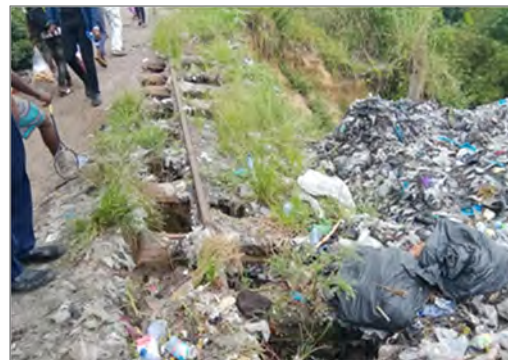
Figure 4-24 Embankment Collapsed behind Garbage Dump (Approx. 9 k 400 m from Limete Station)
