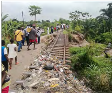
Figure 4-17 Collapsed Embankment (Approx. 5 k 800 m from Limete Station)
