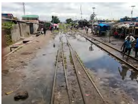
Figure 4-87 Turnout Submerged in Water
