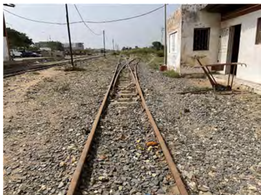
Figure 7-108 Turnout from the Main Line to the Rolling Stock Maintenance Depot
