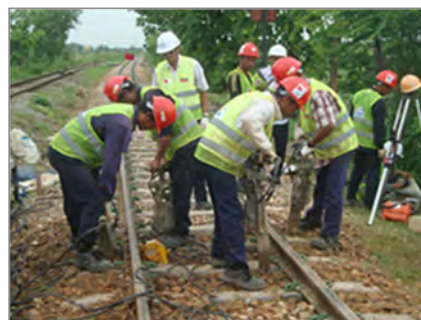
Figure 7-128 Ballast Compacting Work
