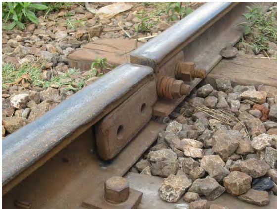
Figure 6-22 Missing Rail Joint Plate Bolt
