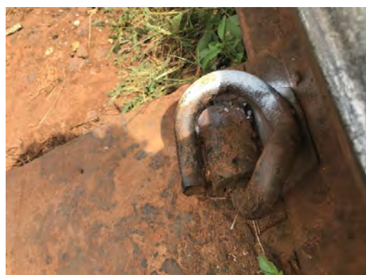
Figure 6-20 Welded Pandrol Clip
