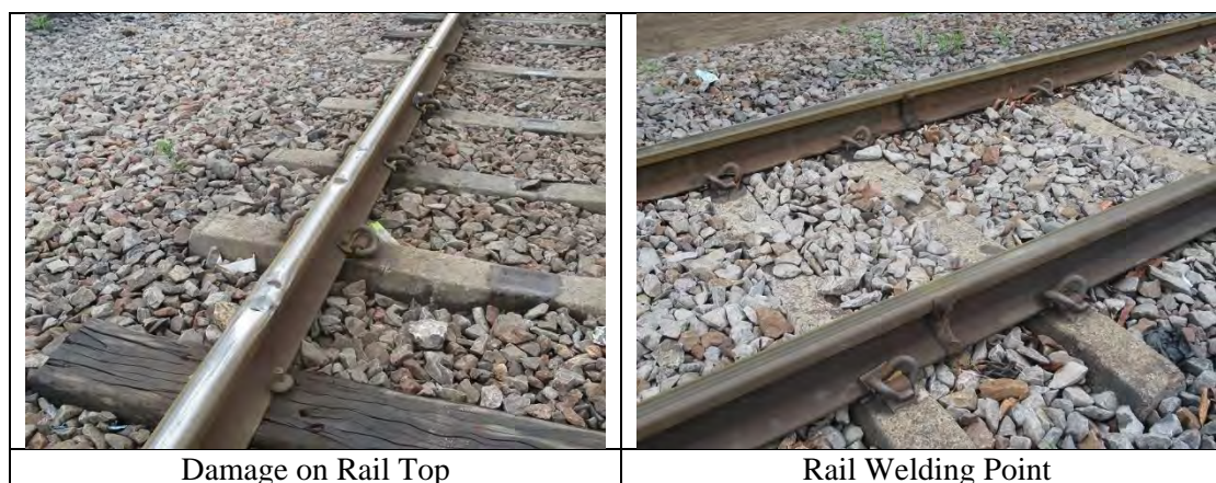
Figure 5-7 Track Condition of Maputo-Matola Gare Rail Line
