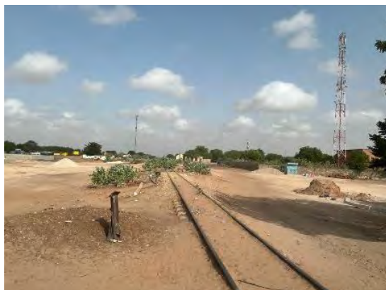
Figure 7-63 Tracks with Sediment Deposits
