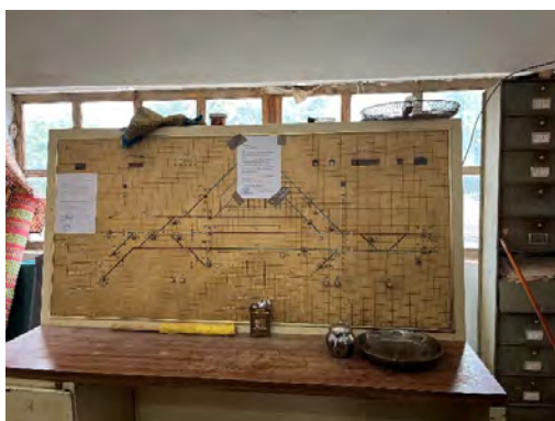
Figure 7-95 Interlocking System at Thiés Station
