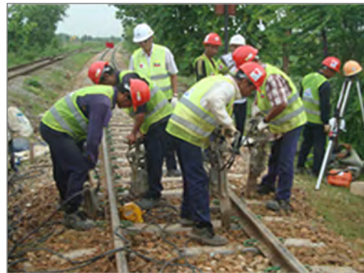
Figure 4-70 Compaction of Ballast
