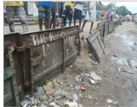
Figure 4-18 Collapsed Steel Retaining Wall (Approx. 6 k100 m from Limete Station)
