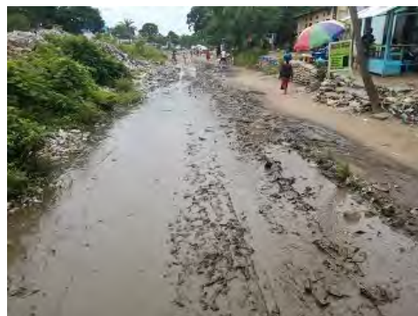
Figure 4-94 Track Submerged by Water is No Longer Visible
