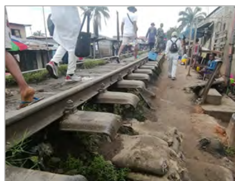
Figure 4-12 Shaved Roadbed/Embankment (Approx. 0.5 km from Limete Station)
