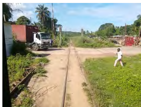
Figure 4-96 Level Crossing Without Level Crossing Plates
