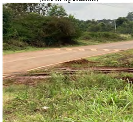
Level Crossing without Warning Device
