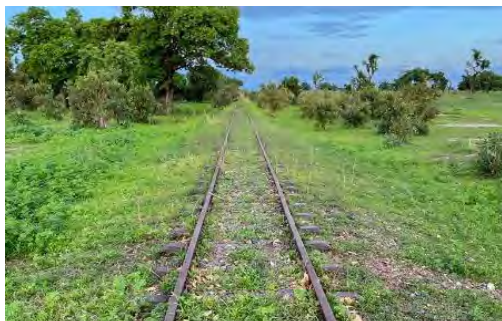
Figure 7-67 Route with Low Ballast Level
