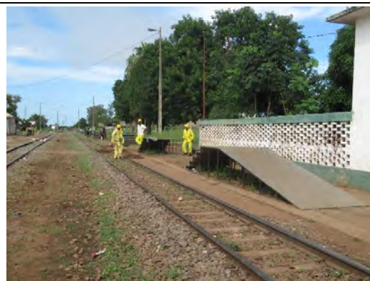
Temporary Steps for DMU Trains
