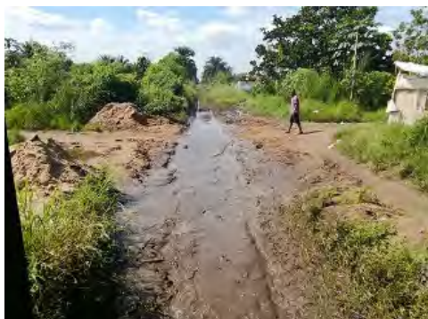
Figure 4-93 Track Submerged by Earth and Sand
