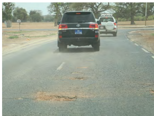
Figure 7-31 Deteriorated Road Pavement
