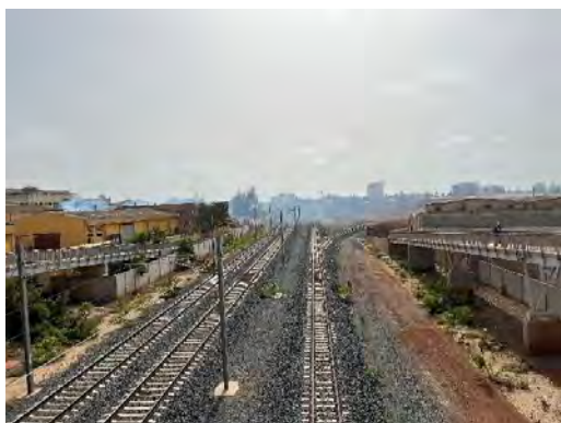
Figure 7-61 Meter-gauge Track Next to the TER Track
