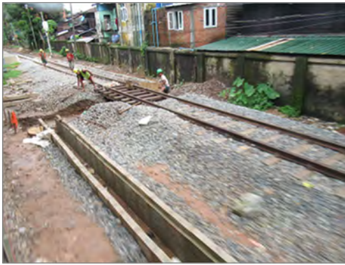
Figure 4-71 Construction of Drainage Channel
