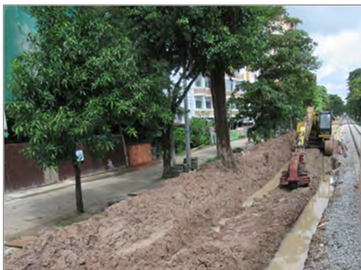
Figure 4-65 Example of Roadbed Maintenance
