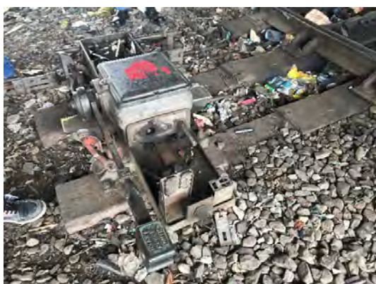
Figure 6-18 Vandalized Electrical Switch
