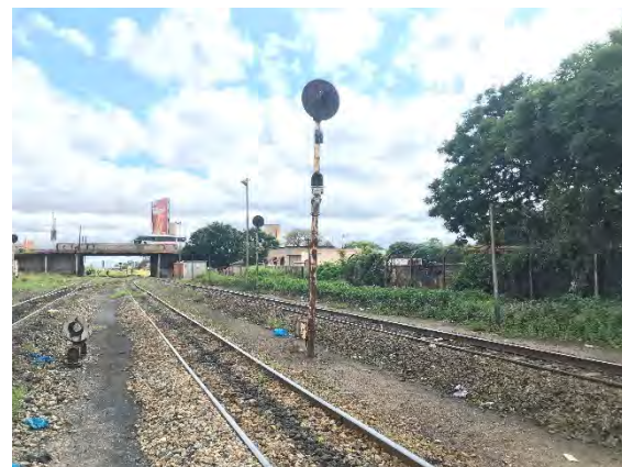
Figure 6-37 Electric Signaling System Not in Use
