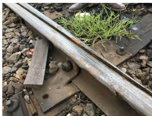
Figure 6-19 Rail Wear
