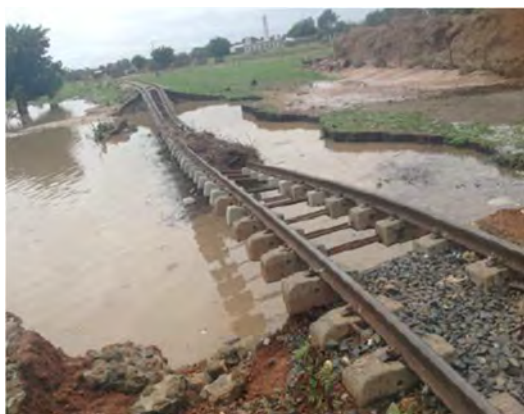
Figure 7-65 Flooded Embankment
