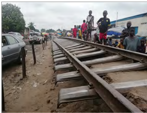
Figure 4-19 Collapsed Track (Approx. 6 k 400 m from Limete Station)
