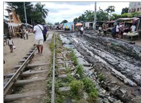
Figure 4-14 Submerged Track (Approx. 1.0 km from Limete Station)
