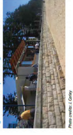
Figure 3-2 Example of a Rigid Vertical Seawall
