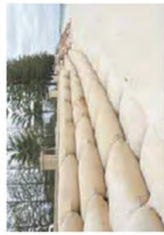
Photo 1: Semi-rigid geotextile container (Maccaferri NZ Ltd.)
