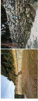
A well-constructed grouted rock wall in New Zealand (left) and informal grouted rock wall in the Republic of the Marshall Islands (right)
