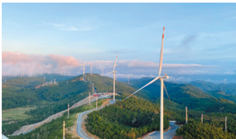
Viet Nam: Under the Private-Sector Investment Finance (PSIF) scheme, JICA co-financed the Quang Tri Province Onshore Wind Power Project along with the Asian Development Bank and Export Finance Australia. The investors are RENOVA, Inc., a renewable energy power producer in Japan; and PC1 Group Joint Stock Company, a power supplier in Viet Nam. The project was completed in October 2021 and the wind farm is now generating power. (Photo: RENOVA, Inc.)
