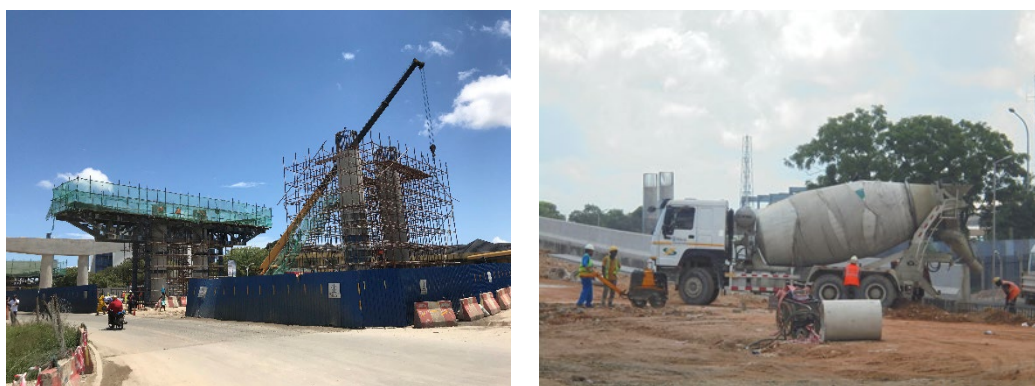
Figure 2-2-1-4.1 Example of construction work
