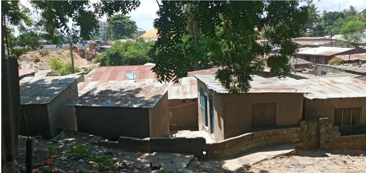
Photo 1: Some of residential structures to be affected at Kibo mtaa in Ubungu ward Source: EARG Study Team, February, 2020
