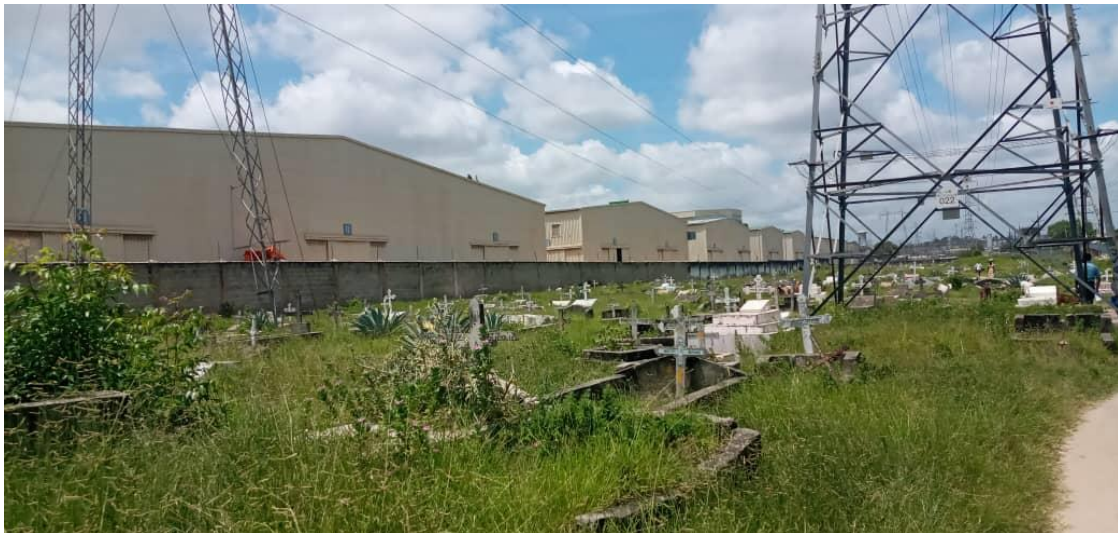
Photo 11: Ubungo Kisiwani Grave yard in the existing Power transmission line likely to be affected by the New transmission line at Ubungo Kisiwani in Ubungo ward
