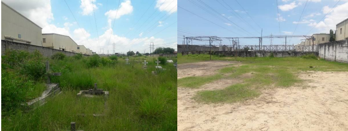
Photo 6: Extended wall within the existing power transmission line at Ubungo Kisiwani
