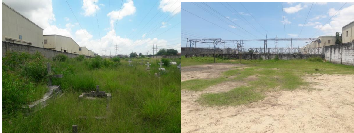
Photo 12: Extended wall within the existing power transmission line at Ubungo Kisiwani Source: Source: Field survey, EARG Team, 2020
