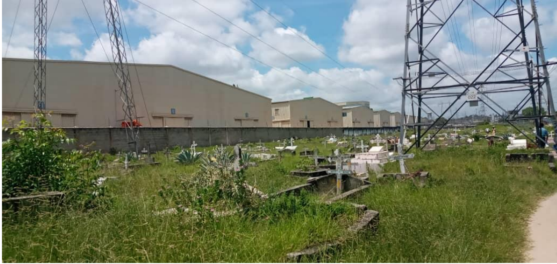
Photo 8: Graves in the existing Power transmission line likely to be affected by the New transmission line at Ubungo Kisiwani in Ubungo ward
