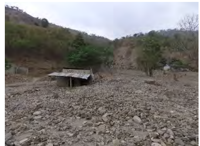
6.1 km (R): House on right bank side is attacked by debris flow.
