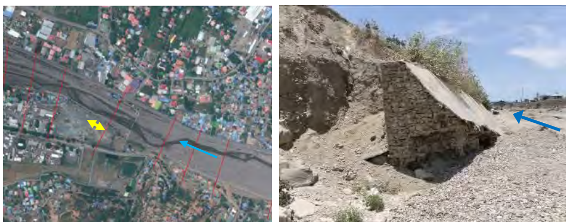
Figure 3.2-18 Damaged Revetment (L2)
