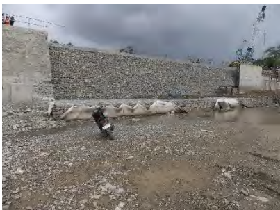
Buluto irrigation: Retaining wall (wet masonry) fell down and urgent recovery was finished.
