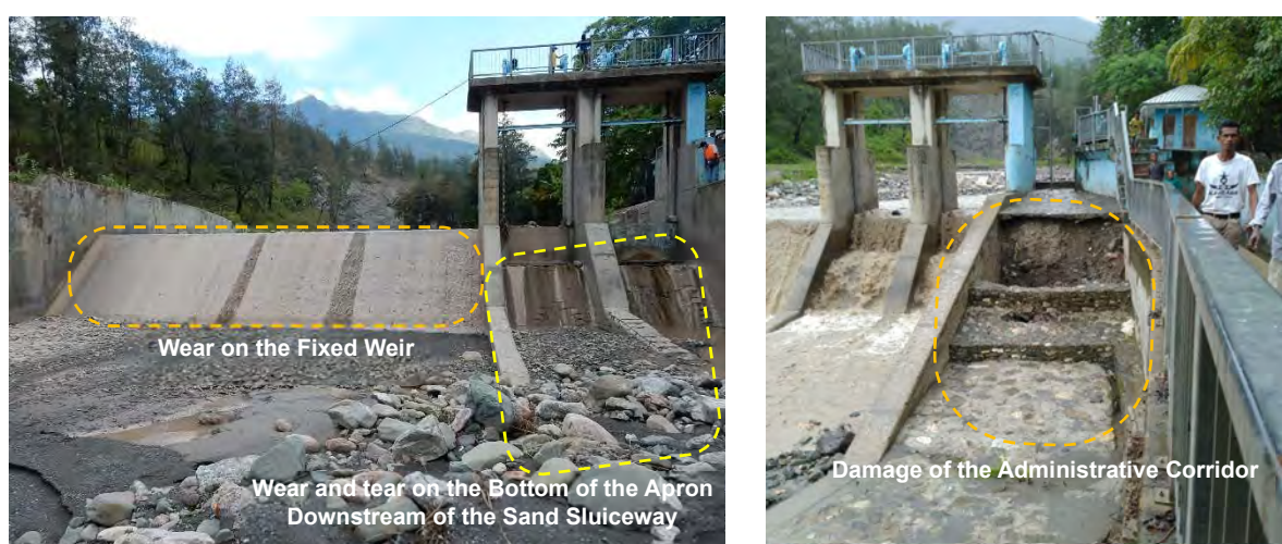
Fig. 3.4-10 Damage on the fixed weir, downstream apron of the sand sluiceway, and administrative corridor in Mariana headworks
