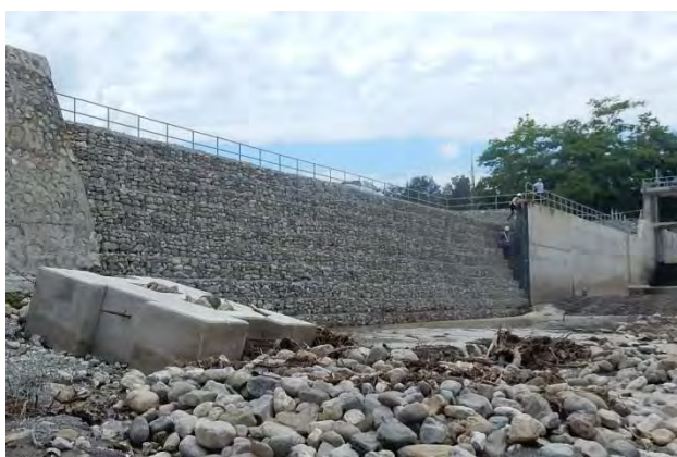
Figure 3.4-5 Temporary Gabion in the collapsed section
