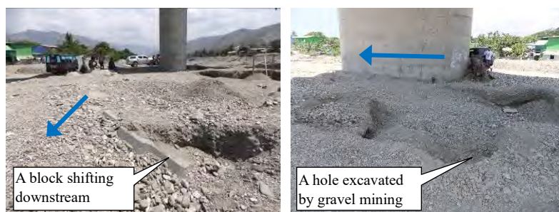
Figure 3.2-30 Riverbed around P3 pier
