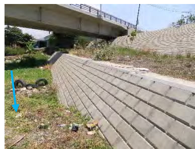
Figure 3.2-3 Revetment of Hinode Bridge
