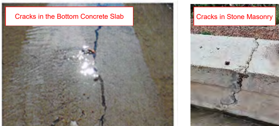
Fig. 3.4-9 Cracks in the cross section of the rectangular canal
