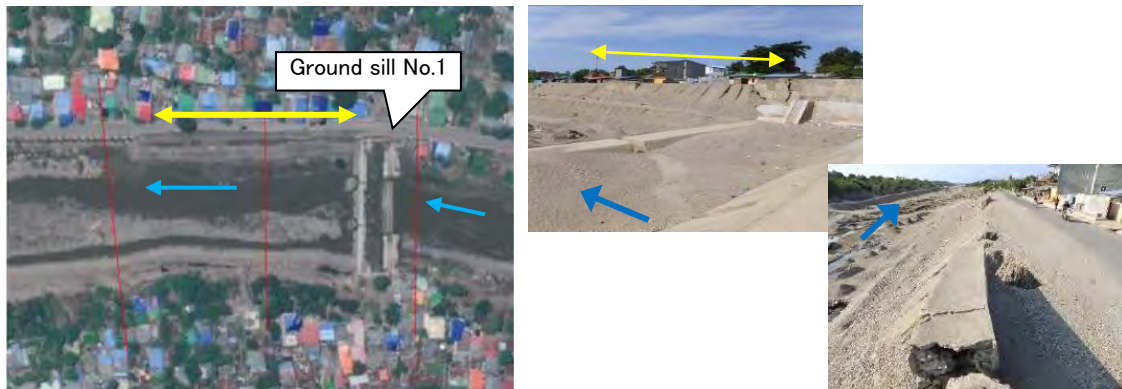
Figure 3.2-21 Damaged Revetment (R4)
