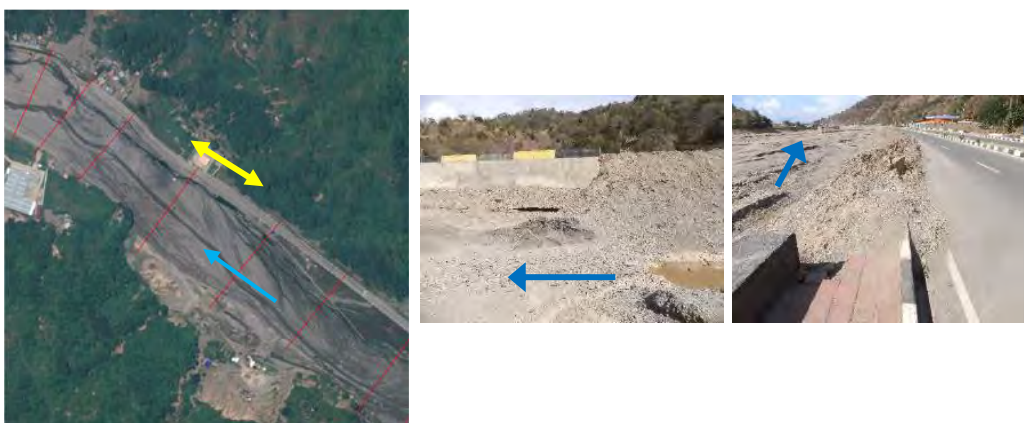
Figure 3.2-27 Damaged Revetment (R10)
