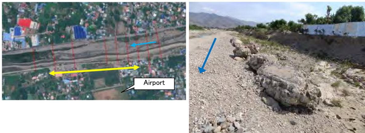
Figure 3.2-17 Damaged Revetment (L1)
