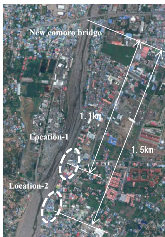
Figure 3.6-2 Fallen location of the Comoro revetment
