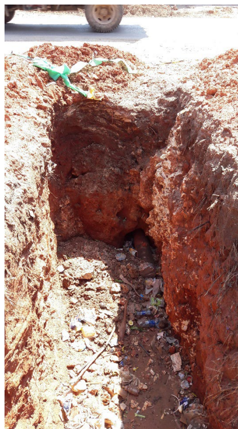
Condition of On-going Pipe Laying Work
