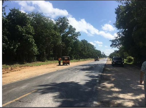
National Road NR-A14 (Main Transmission Pipeline will be installed by the road)
