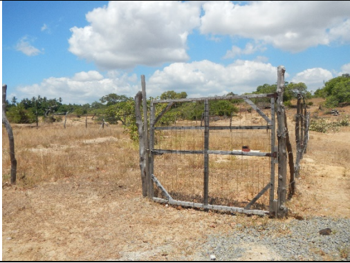
Current Status of Intake Well
