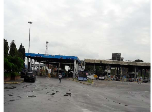
Existing Control Gate around the Surveyed Area
