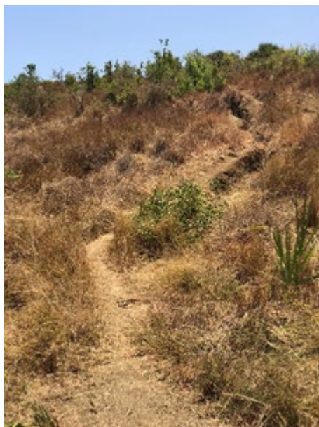
(b) Gully Erosion due to Rain
