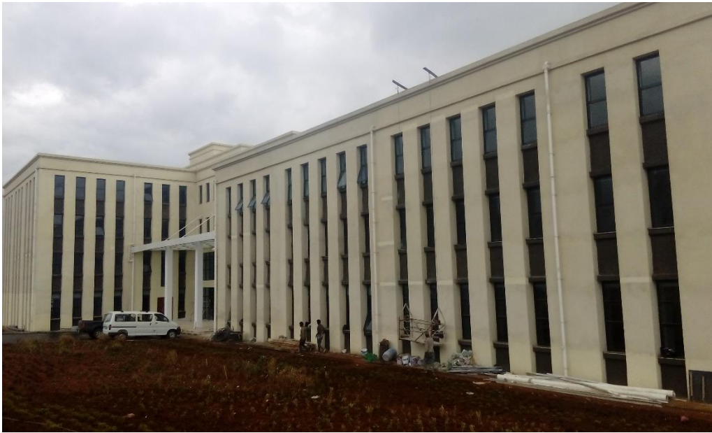
Picture 2. View of the Entrance area
