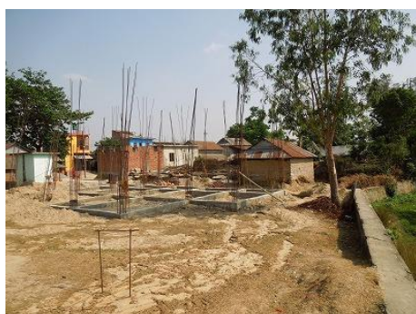
Birth center under construction adjacent to targeted CUP-02
