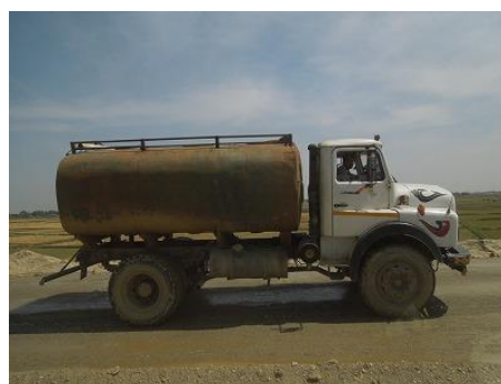
Example of surface watering by Postal Highway Project
