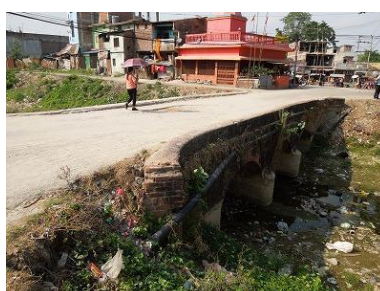
CCB03 (Fiber optic cable: administered by NEA)
