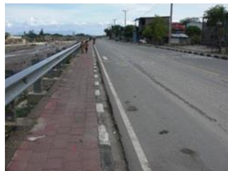
Figure 2-2-5 Existing road conditions
