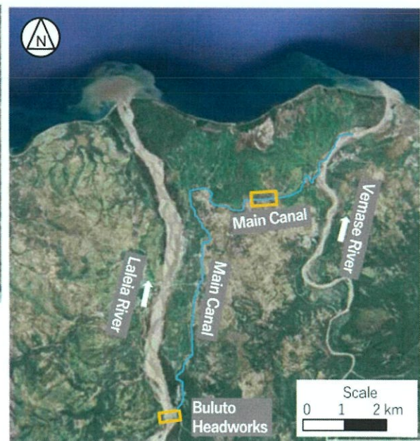
Buluto Irrigation Facilities
