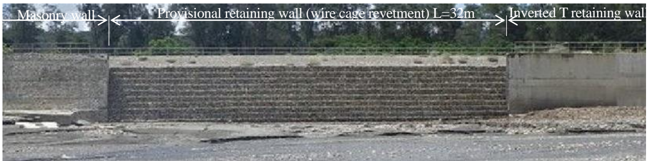
Figure 2-2-26 Provisional retaining wall
