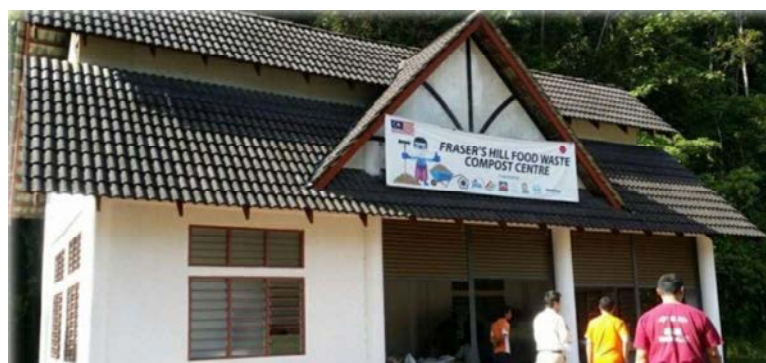
Fraser's Hill Food Waste Compost Centre
