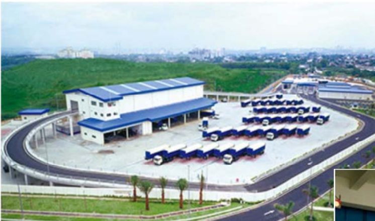
Waste Transfer Station at Kuala Lumpur, Malaysia employing Japanese technologies
