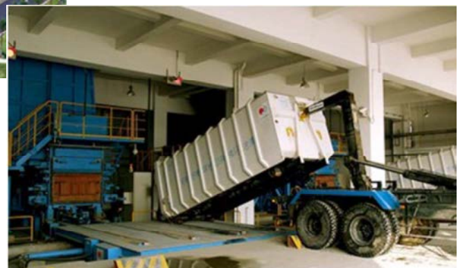
Waste Transfer Station at Xian, China employing Japanese technologies
