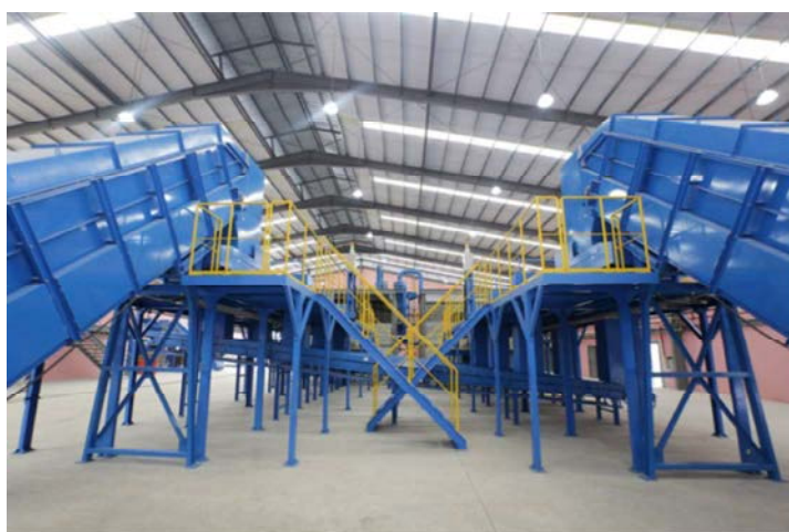
RPF Facility (GUUN's factory in Cebu)
