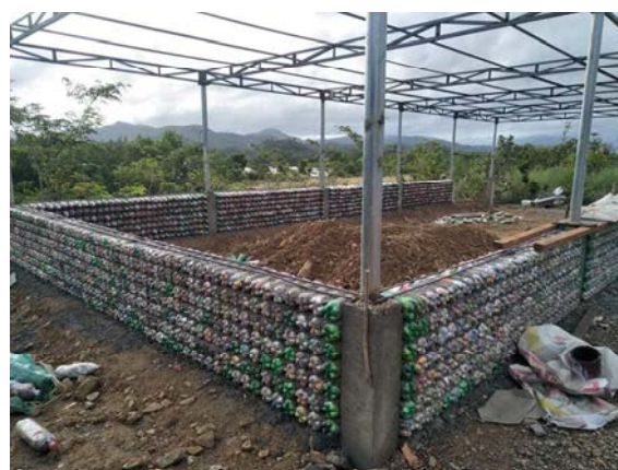
Ecobricks from Ecobricks Philippines used as construction material for fence
