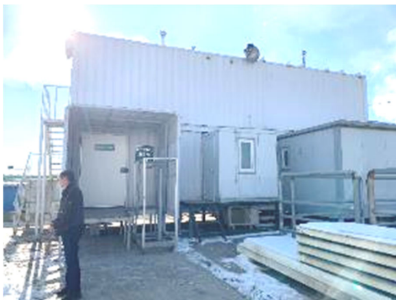
Container slaughterhouse of a private meat company (Precom Ltd)
