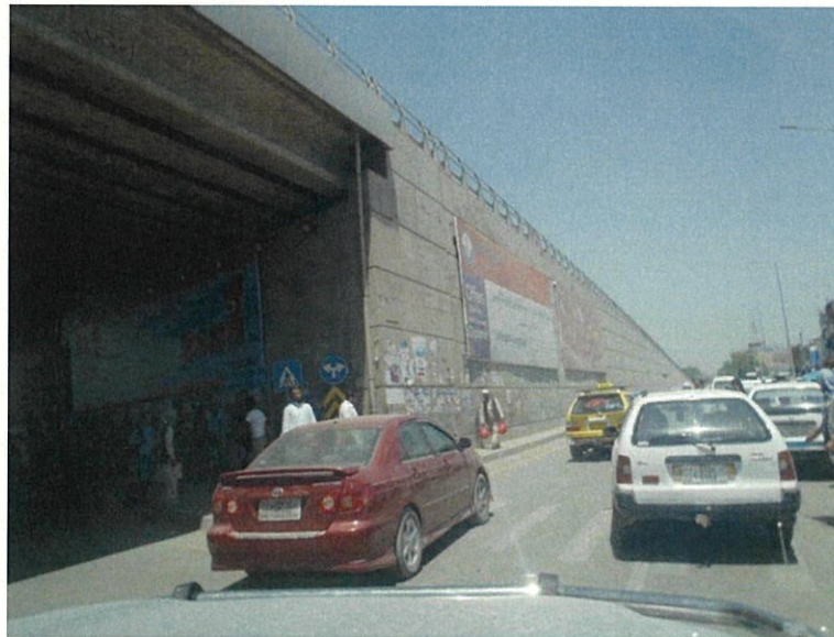
Figure 2-3 Mechanically Stabilized Earth Type retaining wall in Kabul
