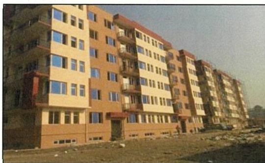
Figure 4-6: Photos from D15-4 (Phase-1) (Source : KM)
