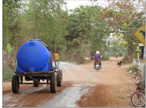
Water sprinkler trucks temporarily reduce dust. (BMC-7)
