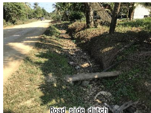
Figure 3.2-45 Road Drainage Facilities
