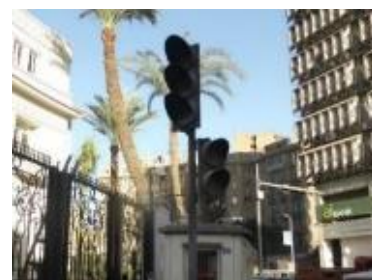
Source: Practical Technology on ITS, JICA Figure 4-12 Broken Traffic Lights
