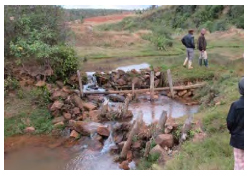
Figure 4 Masonry-Type Traditional Weir (Amaron'i Mania Region)
