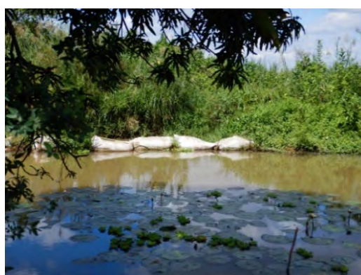
Figure 4 Intake Weir Made of Sacks at Traditional Irrigation Schemes (Morogoro Region)
