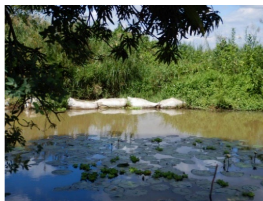
Figure 6.4.3 Intake Weir Made of Sacks at Traditional Irrigation Schemes (Morogoro Region)
