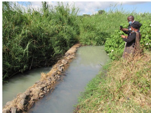
Figure 6.4.2 Intake Weir Made of Stones at Traditional Irrigation Schemes (Mbeya Region)
