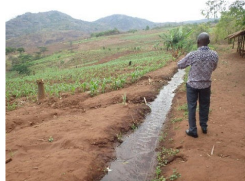
Figure 6.1.2 Simple Weir Irrigation
