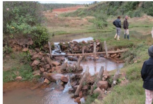
Figure 6.5.3 Masonry-Type Traditional Weir (Amoron'i Mania Region)
