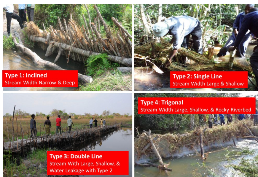
Figure 1.5.2 Four Types of Simple Weir (Zambia)
