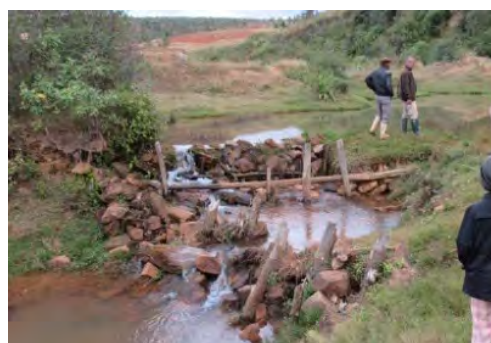
Figure 4 Masonry-Type Traditional Weir (Amoron'i Mania Region)
