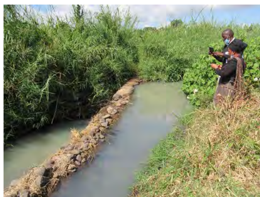
Figure 3 An Intake Weir Made of Stones at Traditional Irrigation Schemes (Mbeya Region)
