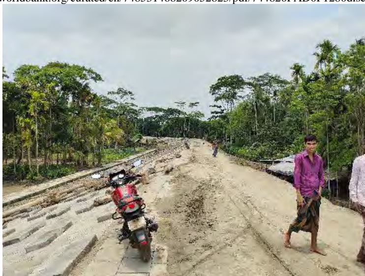
Figure 4.4.7 Storm Surge Bank Under Construction (Polder No.35/1)
