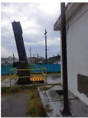
Figure 38 – Location of pump well and column swivel arm (for pump removal and maintenance)
