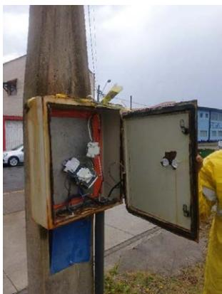
Figure 31 - Improvised closed panel: presents an advanced stage of corrosion and an improper closure with road signaling tape.
