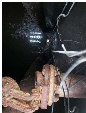
Figure 6 - Non-drowning horizontal centrifugal sewage pump. Below the engine, there is liquid leakage, seemingly sewage, and the metal base of the pumps are in the process of rusting.
