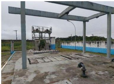
Figure 14 - Overview of the pumping station. In the background: generator house and in the front the top view of the suction well slab with the air inlet and outlet system and concrete covers. There are gaps between the covers, as one of the covers fell into the well.
