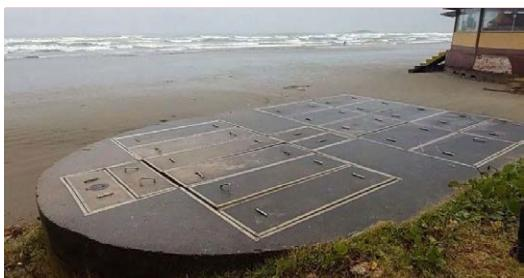
Figure 30 - Improvised open panel. The original panel installed was carried away by the tidal.
