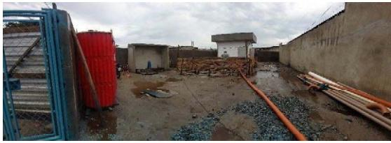
Figure 44 - Pump well under construction. The pressure pipe has been installed, as well as the gate.
