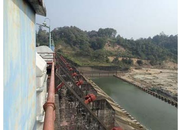
2020/01/20@Kaptai Dam Spillway Rehabilitation of concrete blocks in downstream of apron
