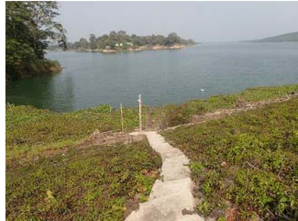
2020/01/20@Kaptai Dam Water level gauge
