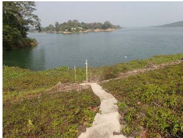
2020/01/20@Kaptai Dam Water Level Gauge
