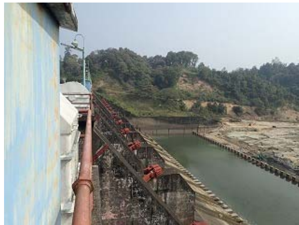
2020/01/20@Kaptai Dam Spillway Rehabilitation of concrete blocks downstream of the apron
