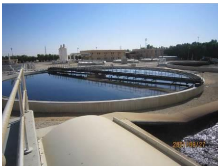
Photo 4-12: Sewage treatment plant near Buraydah
