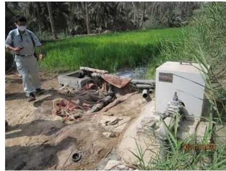
Photo 4-15: Outlet of reclaimed water supply by SIO in Al-Ahasan
