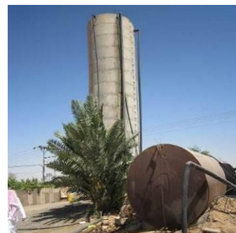
Photo 4-2: Elevated water tank
