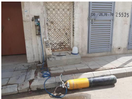
Injection of helium gas into the pipeline
