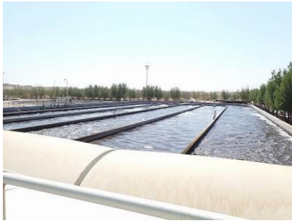
Aeration tank (Carrousel typed oxidation ditch
