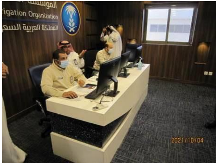
Photo 4-14: Control center for reclaimed water
