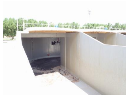
Inside of aeration tank
