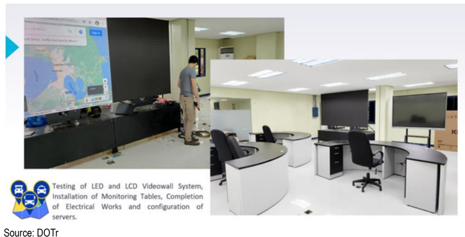
Figure 4.3.2 Central Monitoring Center
