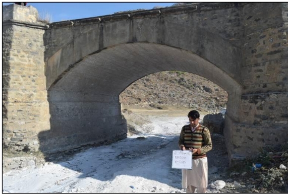
Arch Bridge (No.5 2+448)
