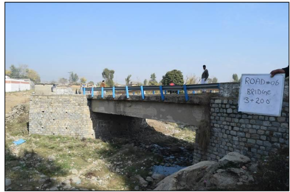
RC Bridge (No.6 Sta. 3+200)
