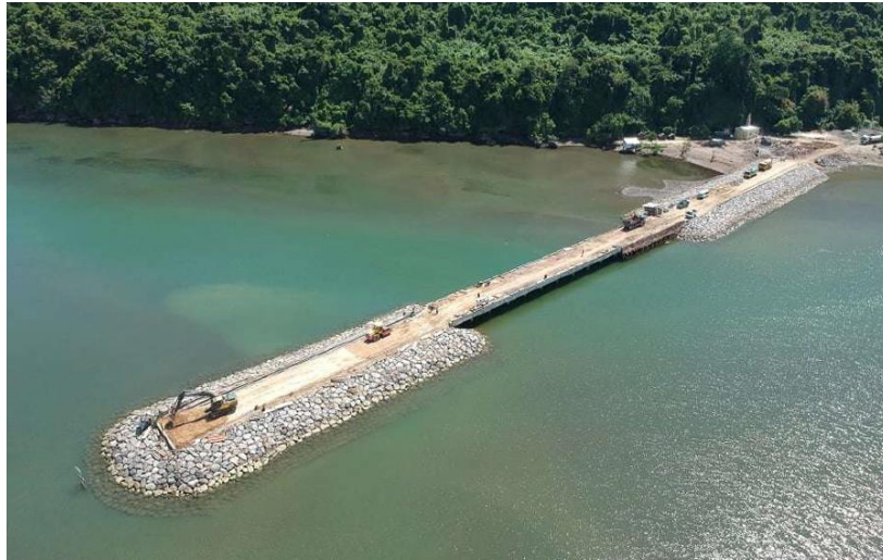
Figure 13.1-4 Construction of Part of Short-Term Development Plan of Timako Port (Under Construction)
