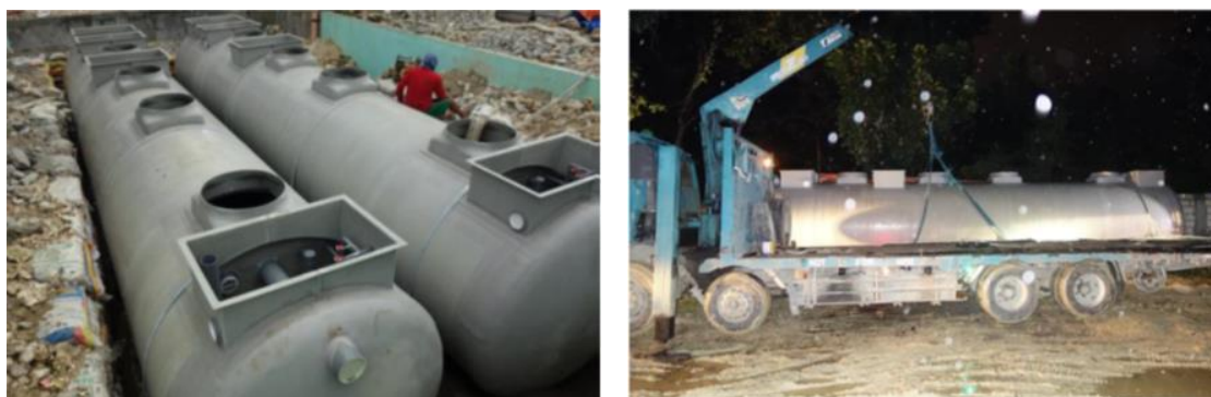
Figure 15.5-8 Example of Installation of Johkaso in the Philippines
