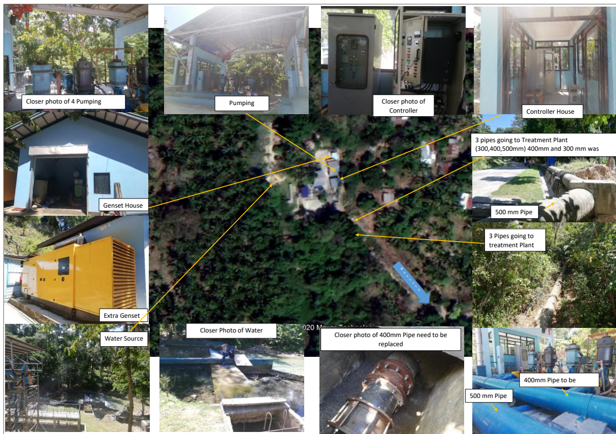
Figure 14.4-8 Photos of Pumping Station in Dimapatoy
