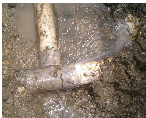
Figure 14.6-3 Image Photo of Water Physical Losses
