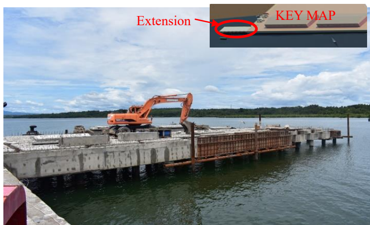
Figure 13.6-1 Extension of 50m of Marginal Wharf
