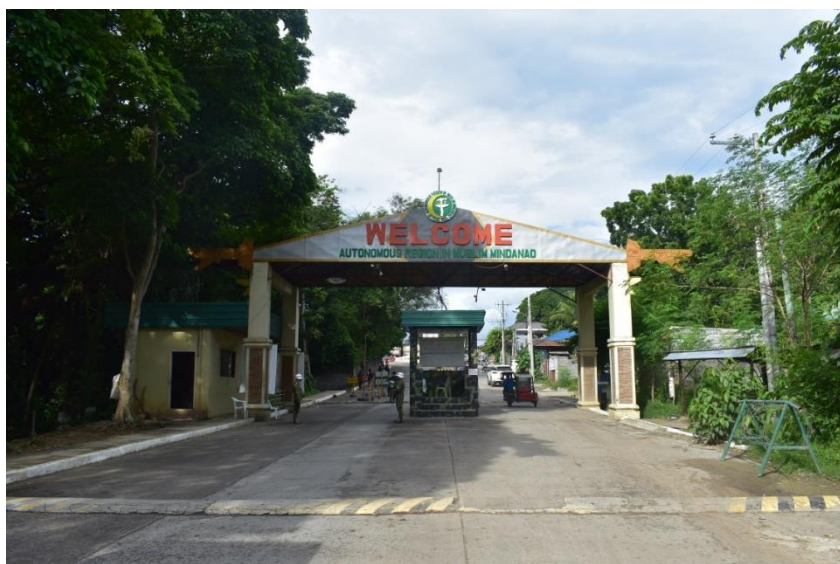
Figure 5.2-13 Access Road with Checkpoint from Awang Airport to National Highway
