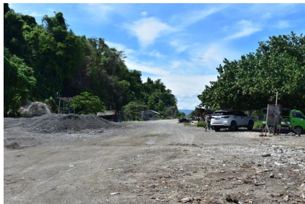
Condition of the of the access road (40m offset)
