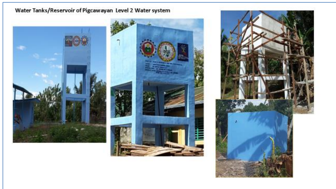
Figure 5.4-19 Photos of the On-going Level 2 Water Projects in Pigcawayan
