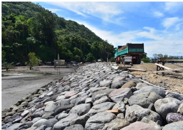
Revetment of Causeway
