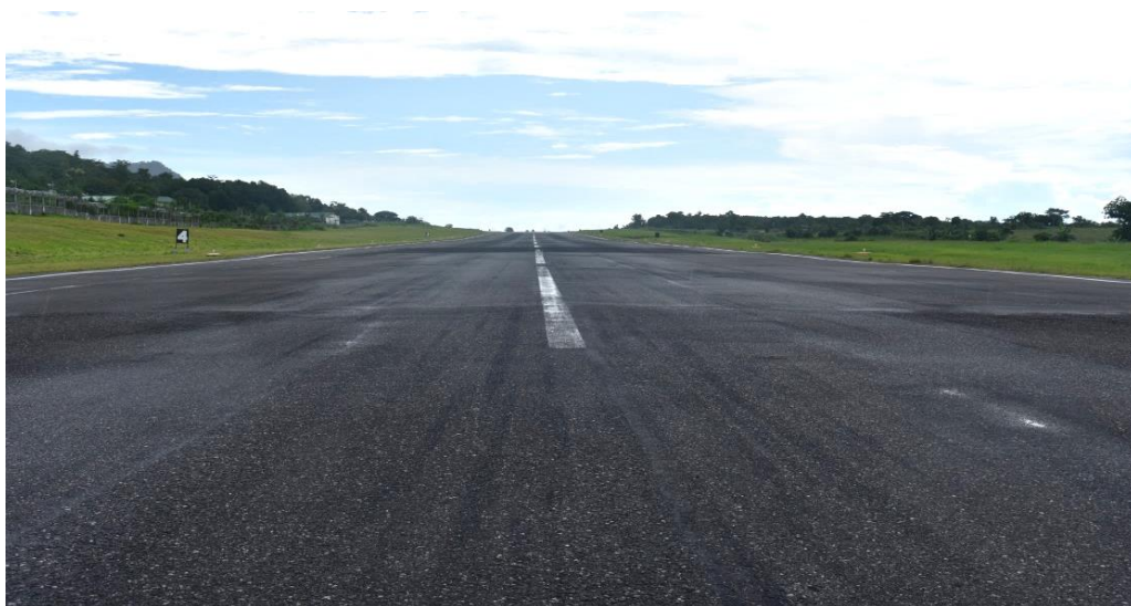
Figure 5.2-3 Middle section of the Runway of Awang Airport
