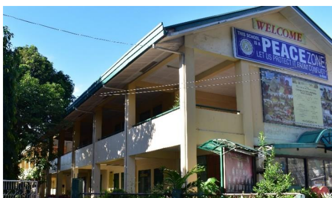
Figure 3.4-5 Photo of a Public School in Cotabato City
