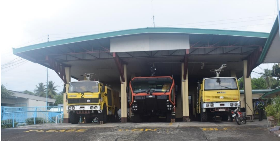
Figure 5.2-10 Aircraft Rescue and Firefighting Facilities
