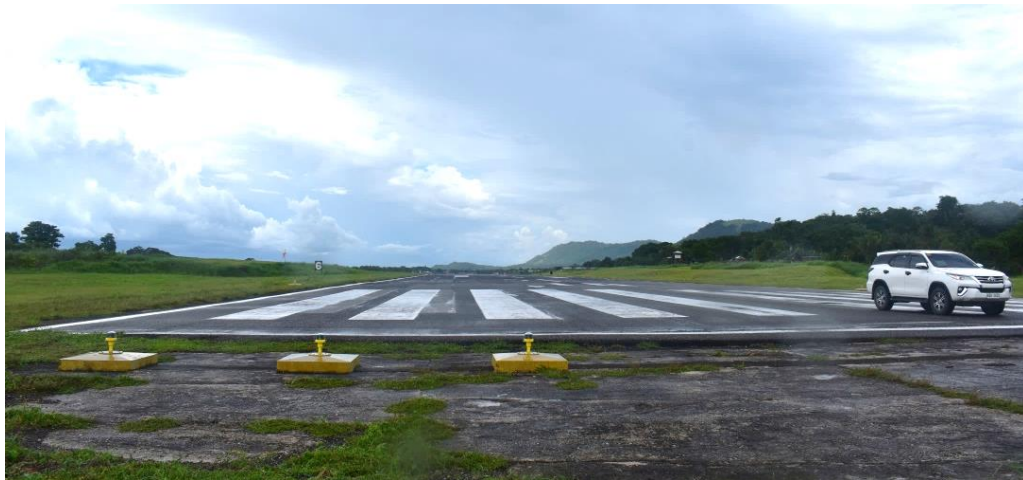
Figure 5.2-2 Runway End No. 10 (western end) of Awang Airport
