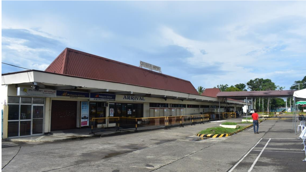
Figure 5.2-6 Passenger Terminal Building of Awang Airport
