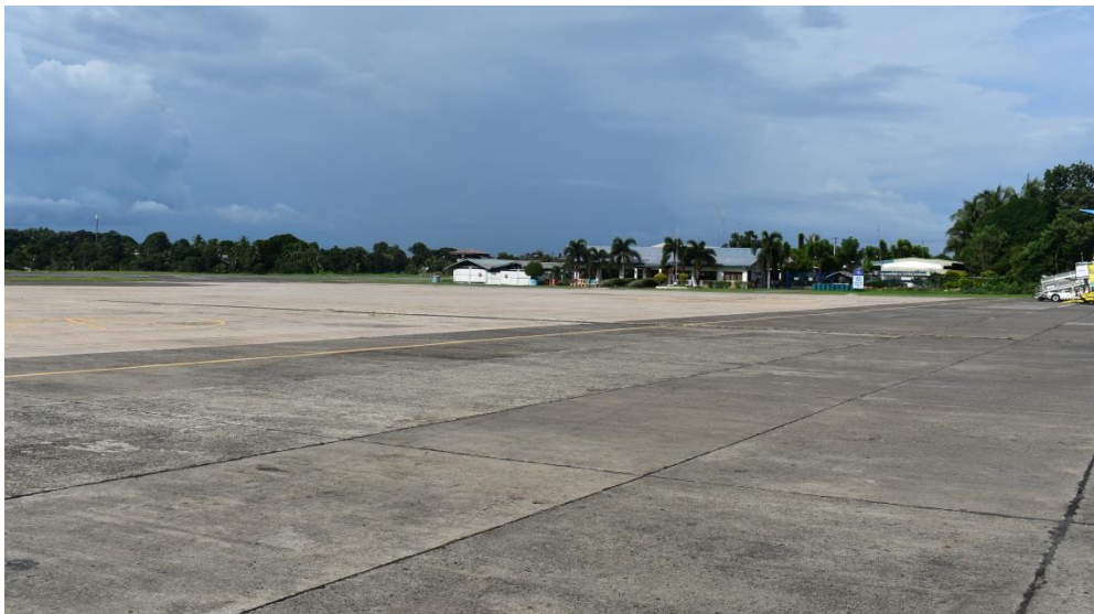
Figure 5.2-5 Apron of Awang Airport
