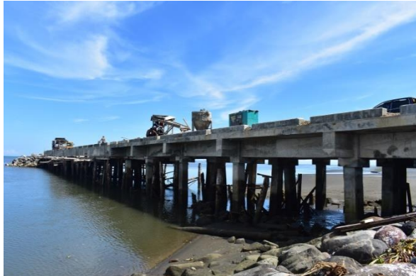
Port Causeway/Trestle leading to the main wharf (29.6m)
