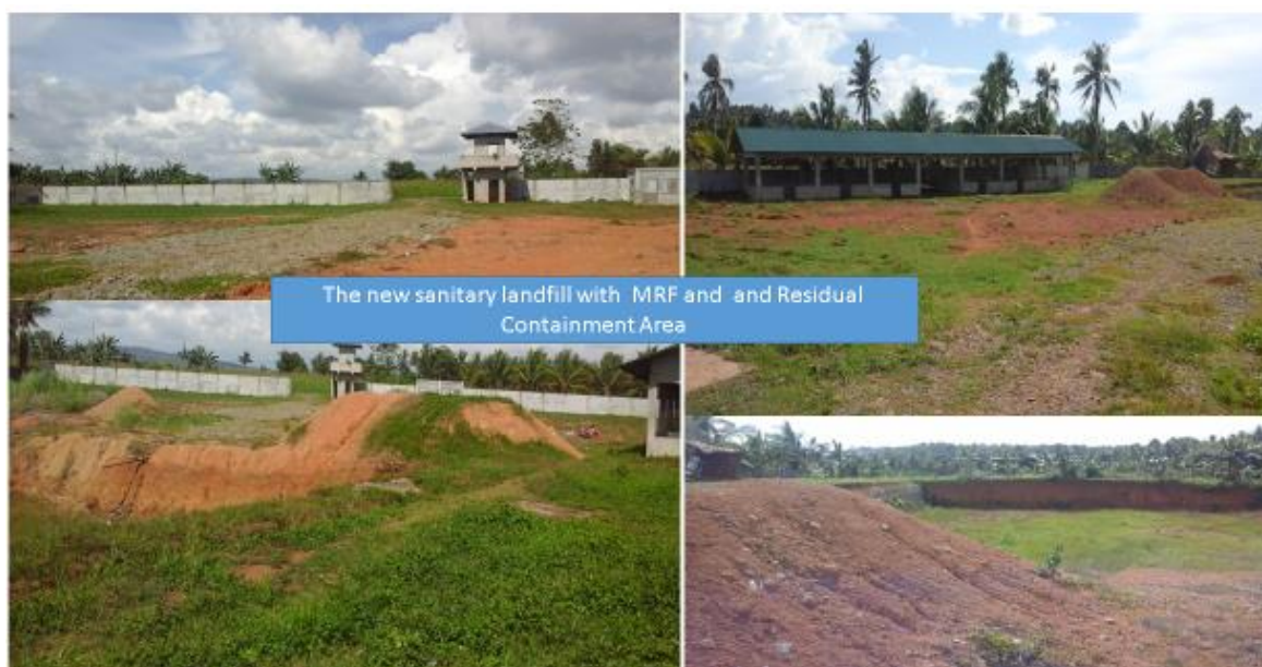
Figure 5.6-7 Newly-developed Sanitary Landfill at Brgy. Gadungan, Parang
