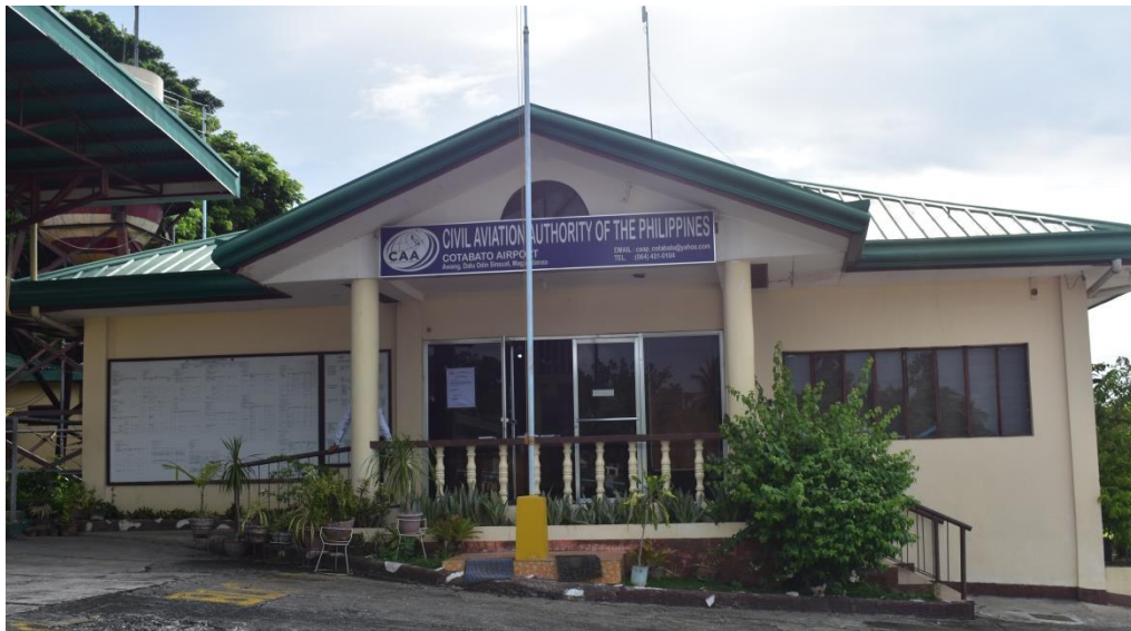
Figure 5.2-9 CAAP Administration and Operations Building
