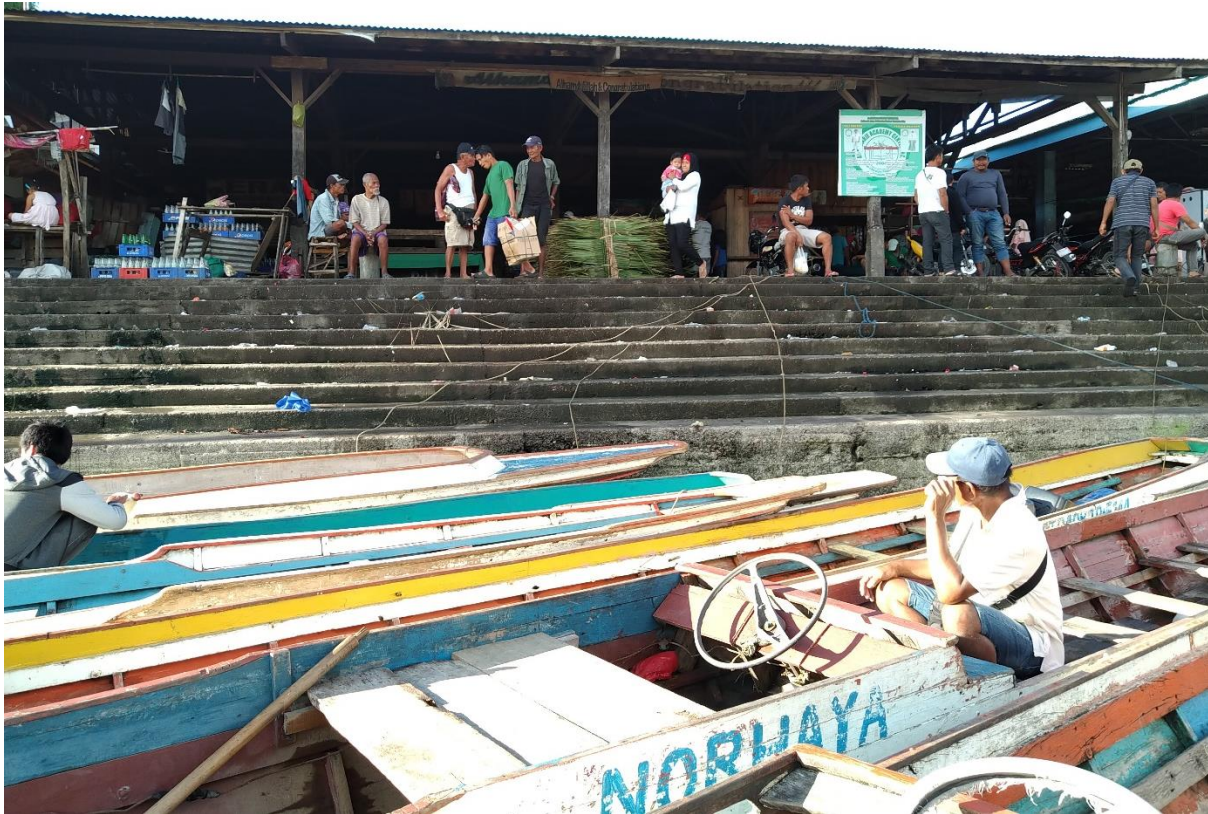
Figure 5.1-22 Photo of the Terminal Building of Water Transport for Inter-city Routes
