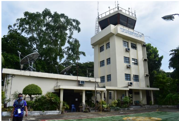
Figure 5.2-11 Air Traffic Control Tower at Awang Airport
