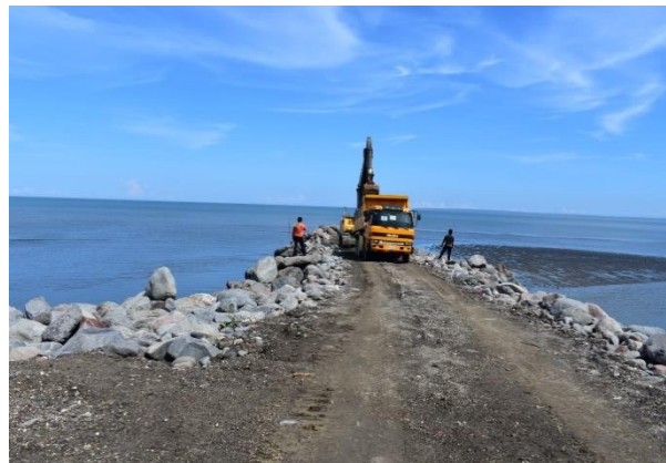
Backfilling of Causeway (On-going)
