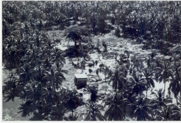
Damage Houses at Seashore of Cotabato City
