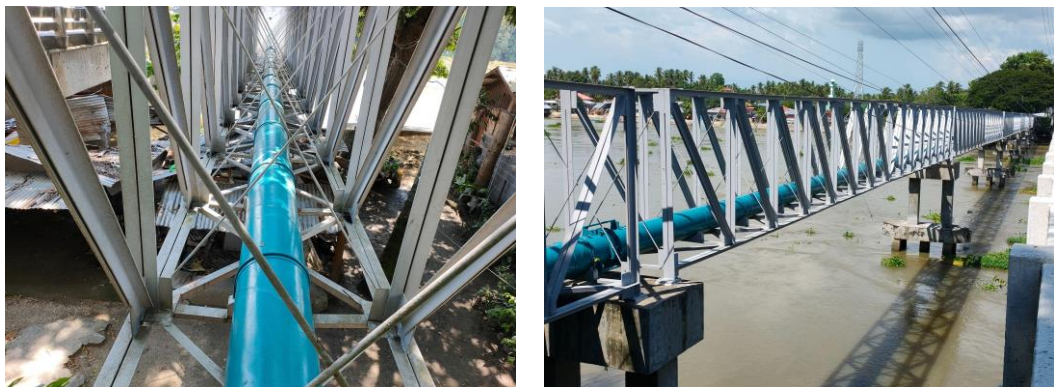
Figure 25.3-6 Existing Pipe Bridge Crossing Tamontaka River
