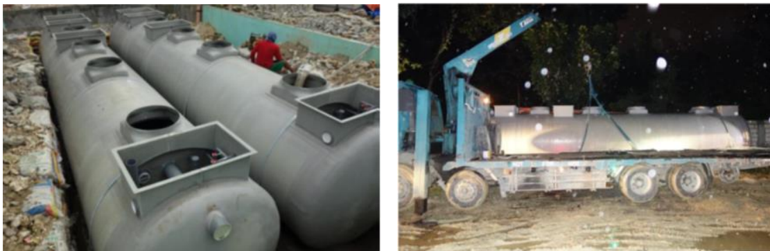
Figure 25.9-8 Example of Installation of Johkaso in the Philippines
