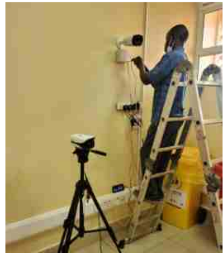
Fixing and calibrating thermo scanner at Mutukula BP
