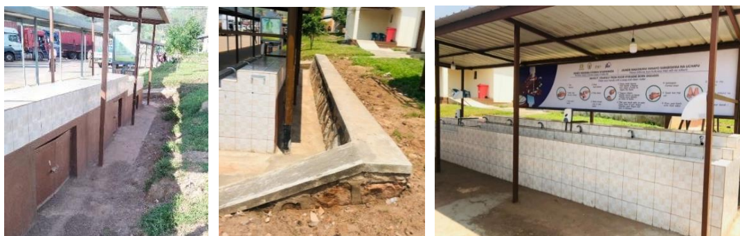
Conditions of handwashing stations at Rusumo BP before pilot activity (left); After refurbishment (centre and right)
