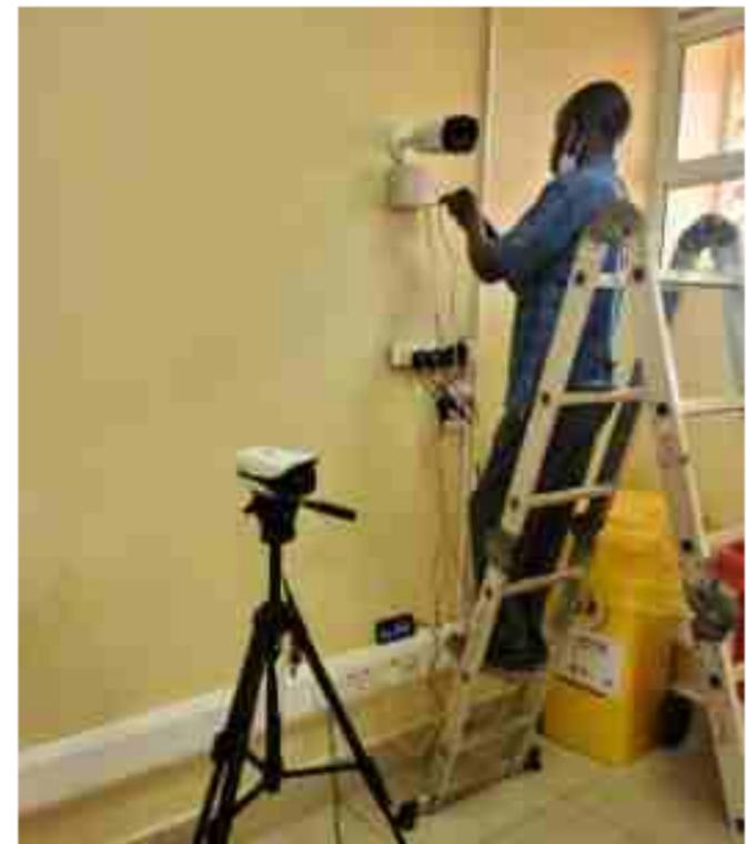
Fixing and calibrating thermo scanner at Mutukula BP
