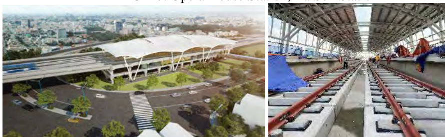
CP2: Elevated Station, Depot
